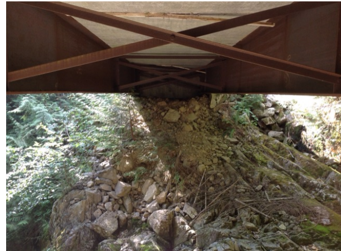
Right Bank Abutment when facing downstream
