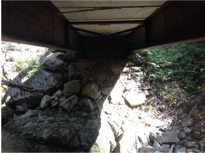
Left Bank Abutment when facing downstream
